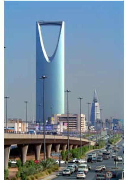
Figure 2: Al-Mamarka Tower — Riyadh
