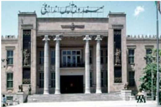
Figure 8: Bank e Melli (National Bank)
