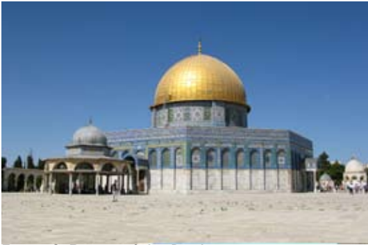
Figure 3: Dome of the Rock
