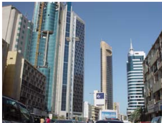
Figure 2: Kuwait's urban environment, a mixture of old and new and tall and short buildings.
